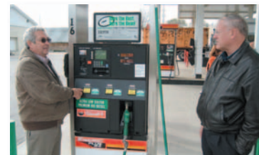
Top: A coordinator presents. Bottom: Hamilton Co-op General Manager Jim Crouch shows Greater New Haven (Connecticut) Clean Cities Coordinator Lee Grannis the biodiesel blending pump (B5, B10 and B20 are offered).
