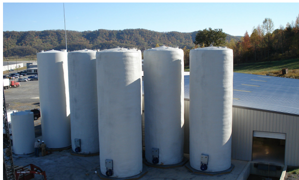
The tank farm at Nu-Energie that holds the raw materials including methanol and the finished product, B100. Truck loading will be just to the right of this picture, and rail access will be just across the street to the left with piping running both raw materials and final product to and from the tanker cars.
